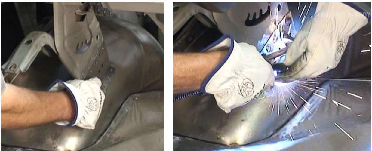
Figure 32 - Fabricate and Weld the Decklid Support
