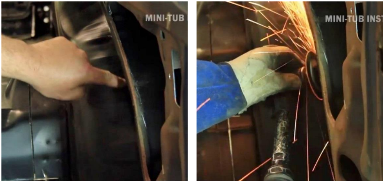
Figure 20 – Cut the Factory Bend Line
