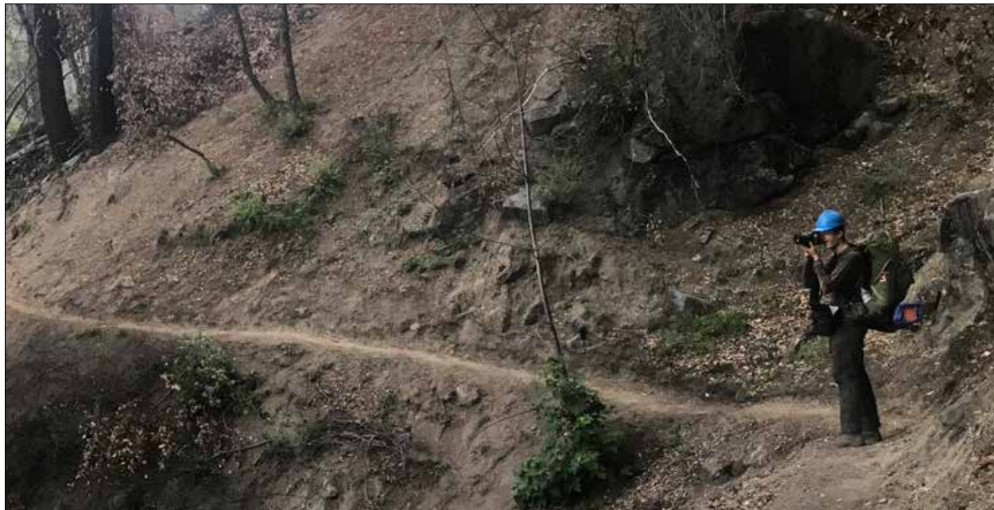
Below: Vincent DiFrancesco documents progress on a newly completed section of the Bridge Creek Trail, Marble Mountain Wilderness. Photo by Nick Hodges.
