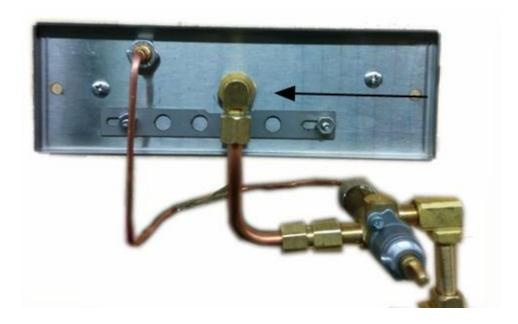
To clean the thermocouple all you need to do is remove the brass wire at the base of the valve. Remove the probe and lightly sand it with scotchbrite or fine sand paper to remove any corrosion. Screw it back into the bottom of the valve ensuring it is tight.
