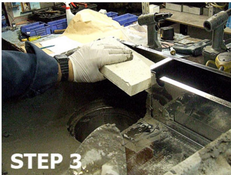
4. And apply cement all around the brick, making sure to fill all the cracks.
