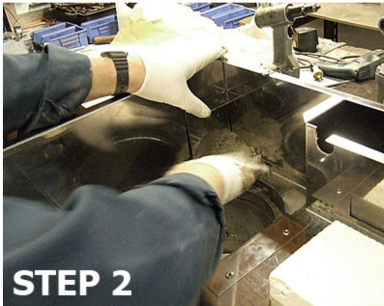
2a. Spread the cement around the stove evenly, about a half an inch thick, and use a trowel to smooth out the surface.
