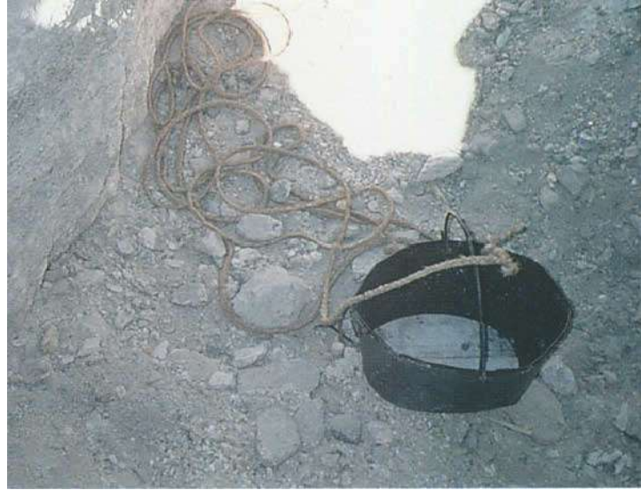
Figure 8c: Bucket to be filled with excavated material and hoisted to the surface on a rope.
