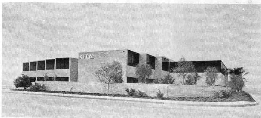
New GIA Headquarters Building, Santa Monica, California
