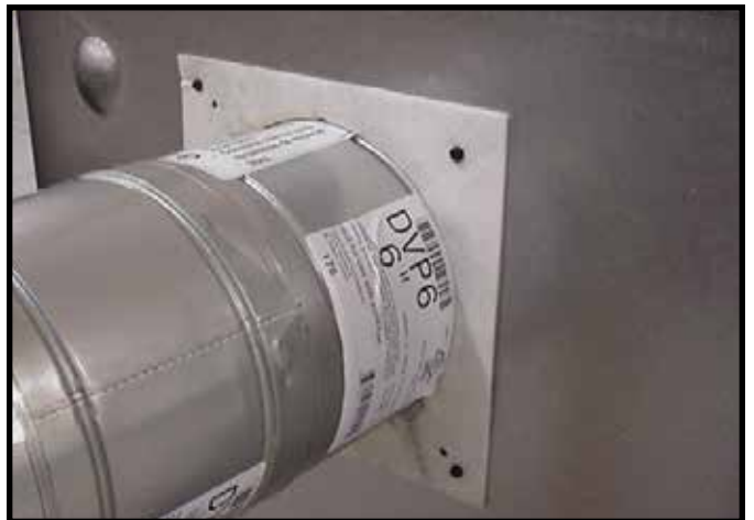
Figure 6.16 (Generic Fireplace Shown) Attach the first vent section (it will snap into place). Slide the insulation gasket onto the vent section, up against the appliance and over the tabs. Use two self-tapping screws to secure gasket to outer wrap.
