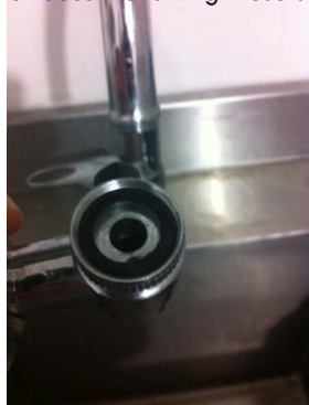
2. Verify the flat gasket is in place in the filter
