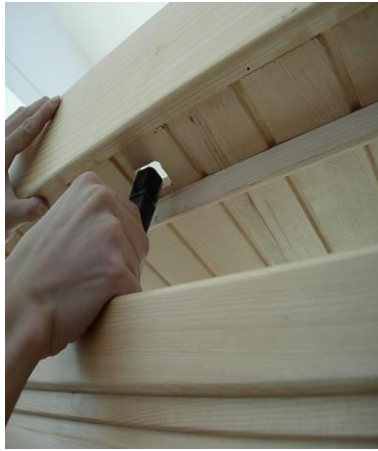
FIG-12 Slip cords/wires through corresponding holes
