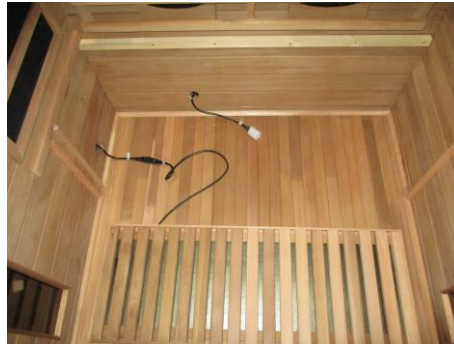
FIG-9 Floor Heater Assembly
