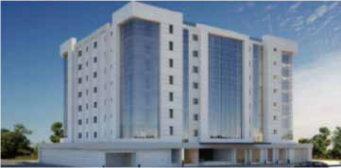
Project Name: Khaled building B+G+7 Project Type: Duct Project Location: UAE
