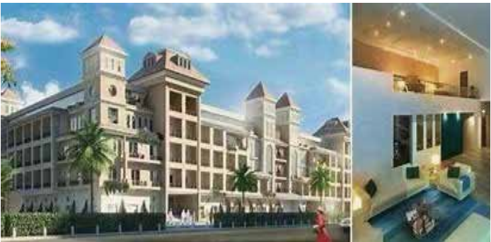
Project Name: Gardenia Residence JVC Project Type: Duct Project Location: UAE
