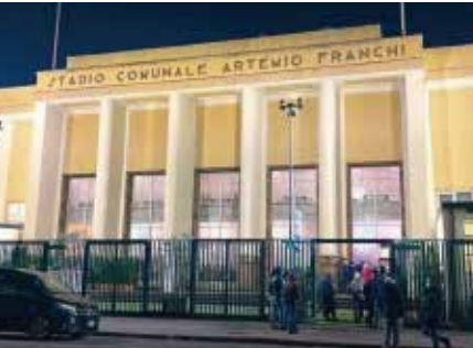
Firenze, Italy. Light Commercial duct and cassette in the restaurant and living areas, RAC in the dressing rooms.
