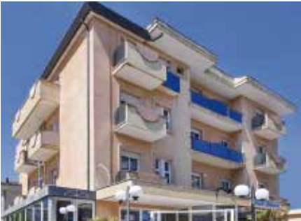
Rimini, Italy. RAC installation mixed with Light Commercial duct and cassette.
