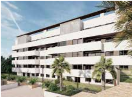
Málaga, Spain. 80 flats developed by Voltiam.
