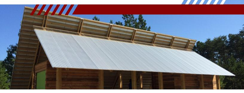
Attached to a building using exposed fasteners, the PBC panel is a popular panel for roof and wall applications in the residential and light commercial markets. This panel is often installed horizontally on walls in commercial applications to provide a contemporary aesthetic.
