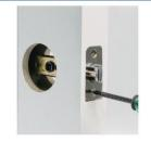
If the latch holes are centered in the door hole, no adjustment is required. Proceed to step 2. If latch holes are NOT centered, adjust latch. See "Latch Adjustment."
