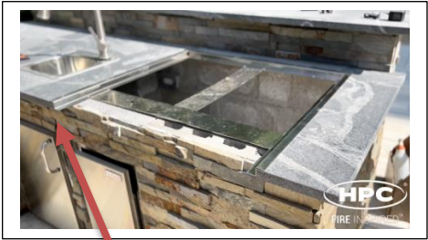
5- Place flange into opening. Edge of flange flush with countertop edge
