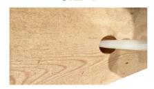
APPLY GENEROUS AMOUNT OF ADHESIVE INTO EACH HOLE PRIOR TO INSTALLATION THIS CREATES A PERMANENT BOND
