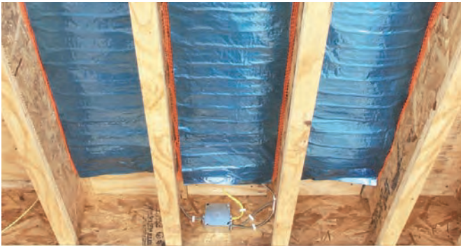
SunTouch UnderFloor - multiple joist bays
