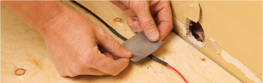
FIGURE 2.23: Secure the cold lead to the subfloor
