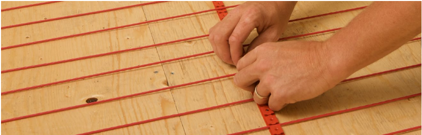
FIGURE 2.29: Install stabilizing guides
