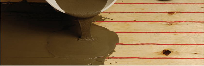
FIGURE 2.42: Self-leveling compound method
