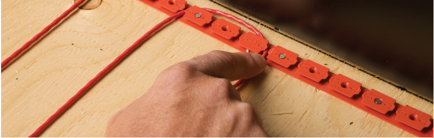
FIGURE 2.26: Install the heating cable
