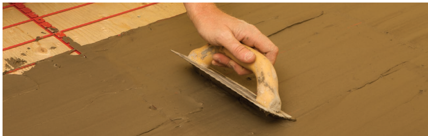
FIGURE 2.52: Thinset mortar method
