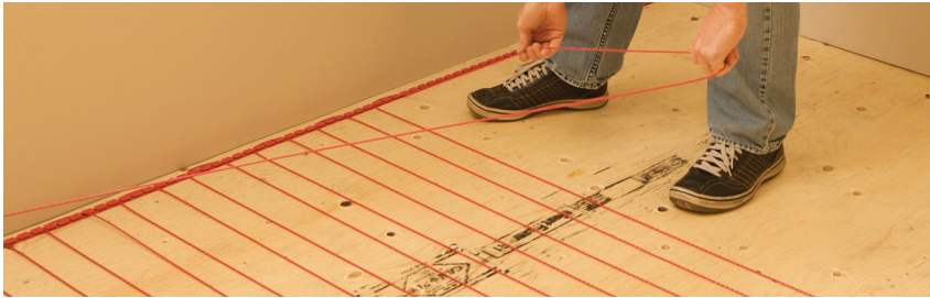
FIGURE 2.27 : Installer le câble chauffant
