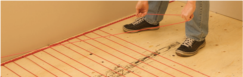
FIGURE 2.27: Install the heating cable
