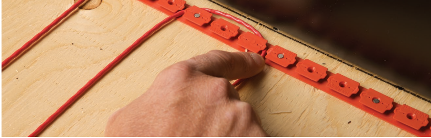
FIGURE 2.26 : Installer le câble chauffant
