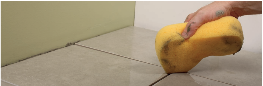
FIGURE 2.23: Clean grout lines
