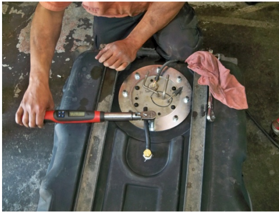
(Fig. 7) Using a torque wrench, tighten the flange nuts to 25 ft. lbs. using a "star" pattern. "Crash Flange" is not shown in this picture.
