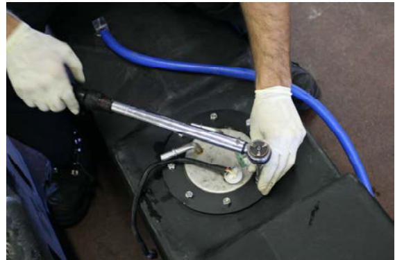
(Fig. 2) Place the sending unit into the TITAN tank, install the top flange, and tighten the nylon lock nuts to 20 ft. lbs using a “star” pattern using a torque wrench.
