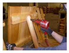
3. Attach angled end of table brace to bottom of table top brace, and be sure to center the brace as much as possible. Use  $2\frac{1}{2}$  lag bolt to secure (as shown).
