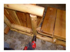
8. Attach swing hangers to arm assemblies using 5" lag bolts.
