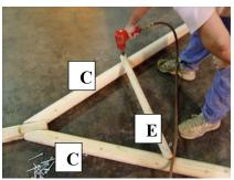
**Step 2:** From machine bolt, measure 32" down swing leg (C), and secure brace (E) using 4" lag bolts and \(^1/4\)" washers. Repeat process for opposite side.
