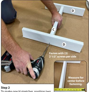
To make one H stretcher, position two 17 1/2" H pieces (D) on their sides as shown above, and place one 18 7/8" H piece (C) on its side and in between them as shown and measure so its centered, fasten with (4) 2 1/2" screws (2 per side) through the pre-drilled holes provided. Make the second H stretcher in the same fashion, with the remaining 3 pieces.
