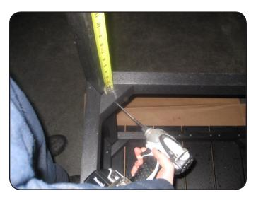
**Step 3** Fasten the leg support assembly (B) measuring 12" to end of legs as shown and fasten from inside with (4) 3" screws (1 per corner).
