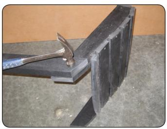
**Step 1**Fasten legs (D) on outside of seat (A) with (4) 3" bolts and nuts.
