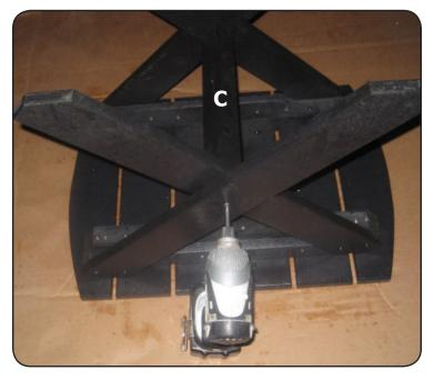
**Step 3**Place the leg support (C) between the legs, as shown. Feed a 3" screw through the holes in the center of one set of legs and into the leg support. Repeat on the other side.
