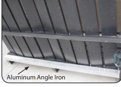
(pictured right), and fasten with (3) 2 1/2" screws through holes in angle iron.
