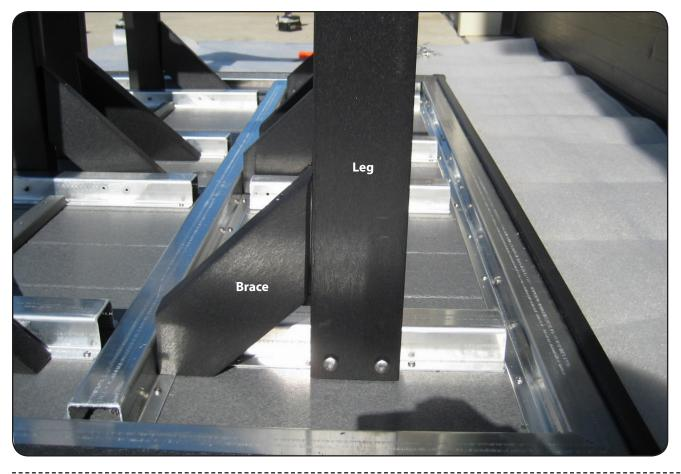
Step 2 Place a brace (C) in between the leg and the angle iron as pictured left. Attach the brace with (4) 1 1/4" screws through the angle iron and (1) 2" screw into the leg. Repeat on the other legs with the remaining braces.
