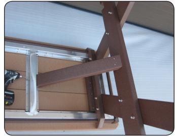
**Step 2**Fasten brace (C) where shown with (8) 2 1/2" screws.
