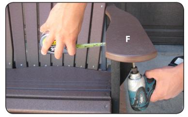
**Step 6**Fasten the left arm rest (F) to side rail in the back with (1) 3" bolt and flange nut. Now measure 1" from inside of leg as shown and fasten on outside with (4) 1 1/4" screws. Repeat with right arm rest on other side.
