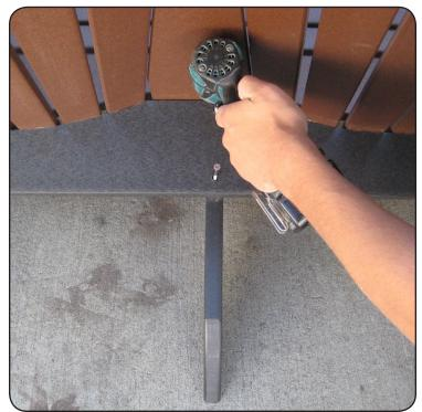
On the back side of the seat, fasten the lower back support to the middle seat support with (2) 2 1/2" Screws through the pre-drilled holes as shown.
