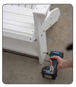
**Step 3**Using (4) 2" screws, attach brace (D) to legs (C).
