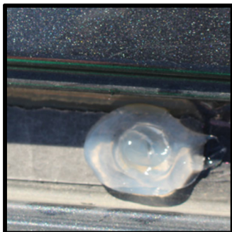
Next apply silicone over the holes
