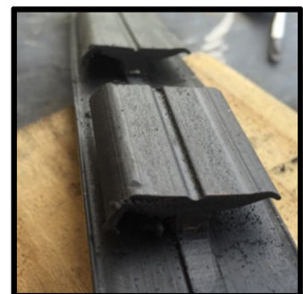
Remove the portion previously cut by making a horizontal cut between the two vertical cuts
