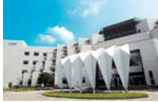
Tainan Plant (Diamond-rated Green Building)
