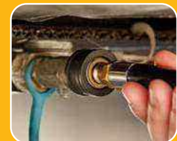
INSERT QUICK CONNECT MALE ADAPTER DIRECTLY INTO FUEL SOURCE
