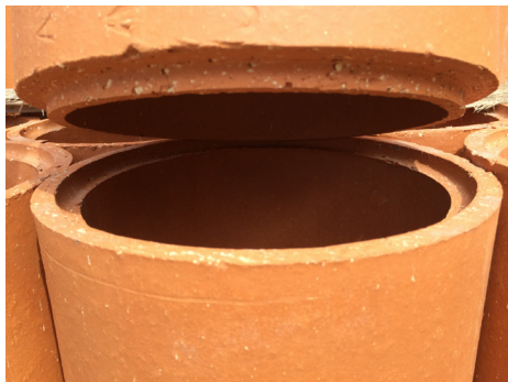
Male/Female End Joints on Round Clay Flue Liners. Male end is always installed down.
