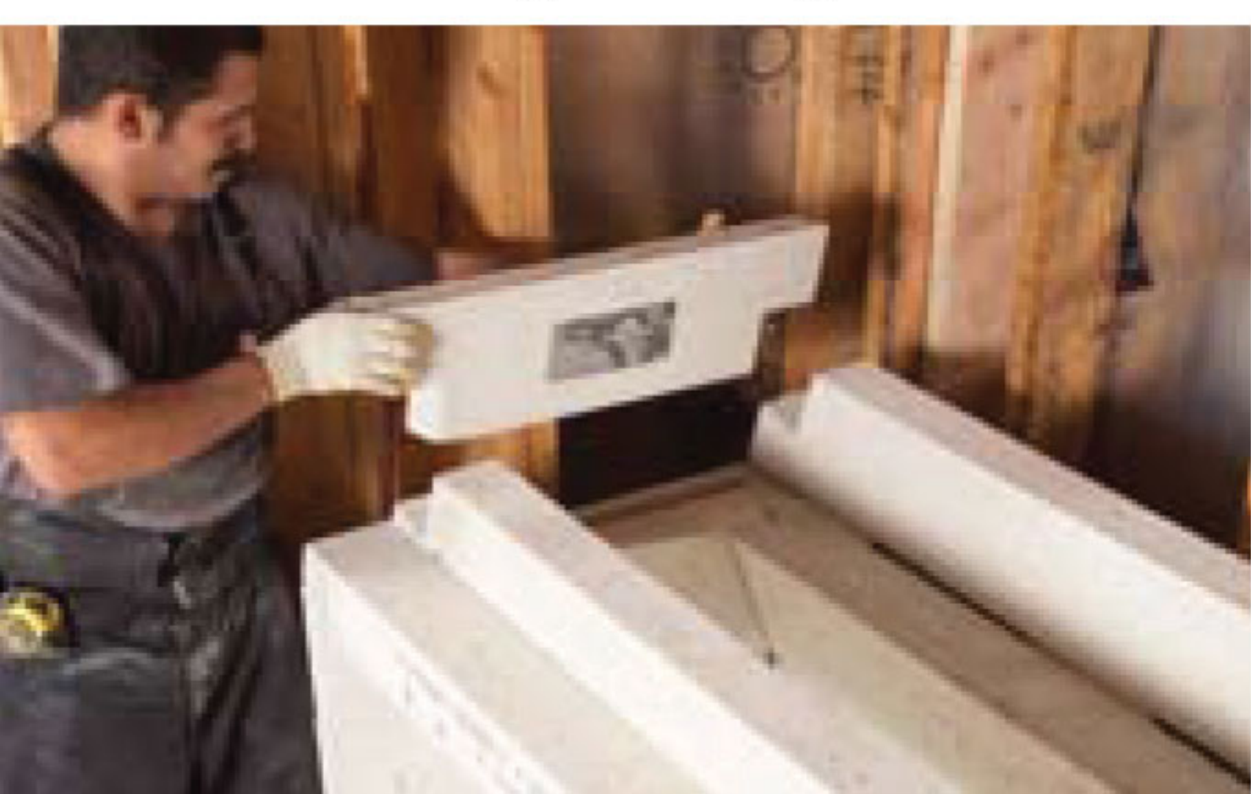
3. Easy to build smoke dome
