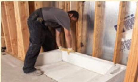
1. Installing base and first course
