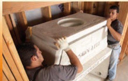
4. Finishing with the dome top
