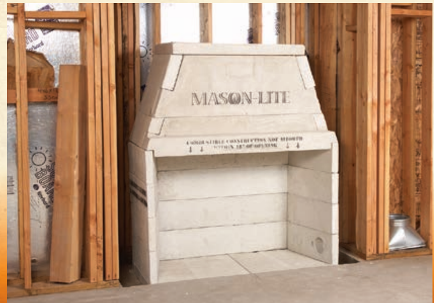
5. Finished Mason-Lite in under 2 hours
