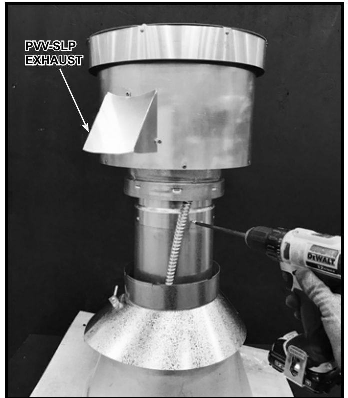
Figure 3.21 Attach PVV-SLP to SLP Pipe
