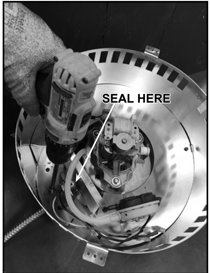
Figure 3.13 Attach Wire Harness Bracket to Bottom Dish
