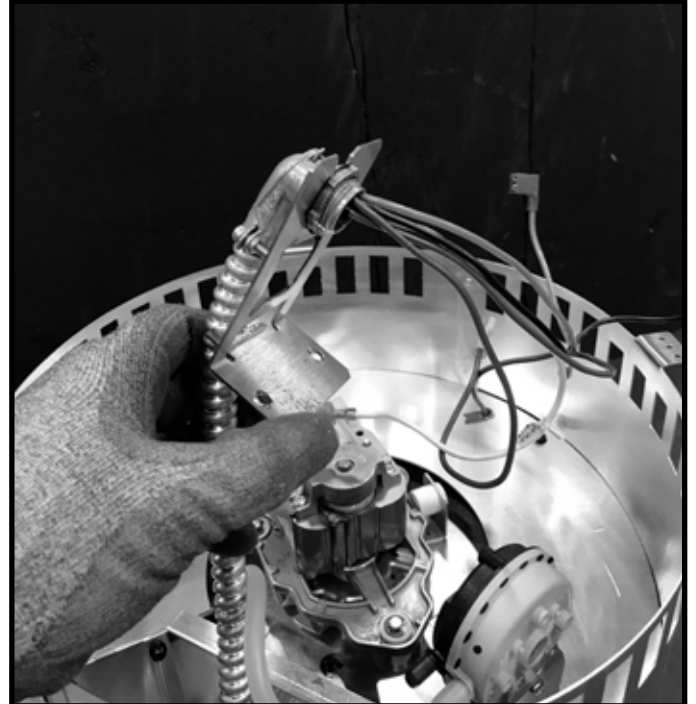
Figure 3.12 Attach PVI Wiring Harness to Bracket
