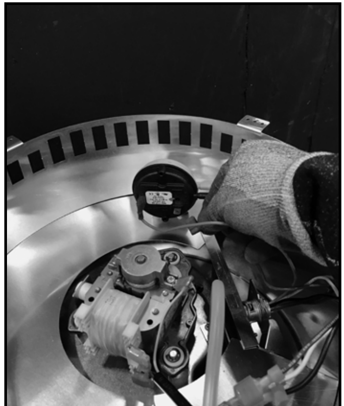
Figure 5.3 Remove Wires from Pressure Switch
