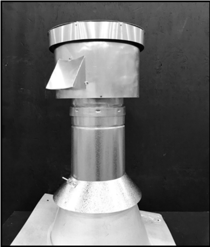
Figure 3.23 Secure Storm Collar in Position on Flashing
