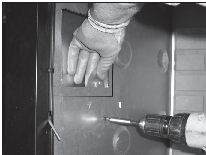
Figure 4 Remove Screw Holding Outside Air Door in Place
