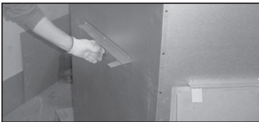
Figure 3.7 Bending Refractory Shipping Tabs Back Down
