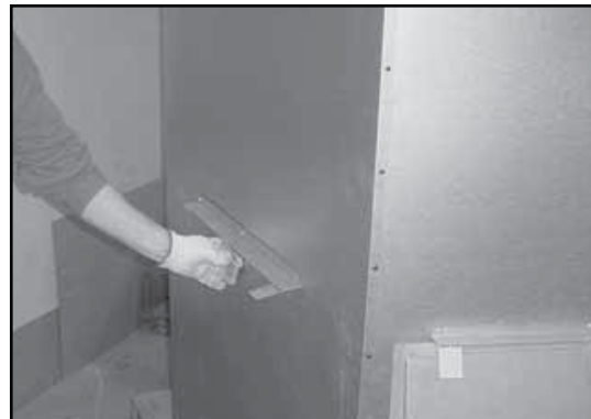
Figure 7.2 Bending Refractory Shipping Tabs Back Down
