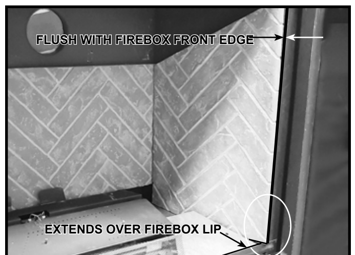
Figure 11.4 Side Refractory Panel Installed (Right Side Shown)
