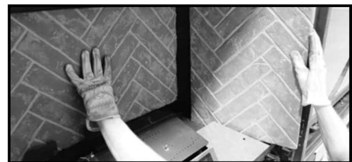
Figure 11.3 Install Side Refractory Panel (Right Side Shown)
