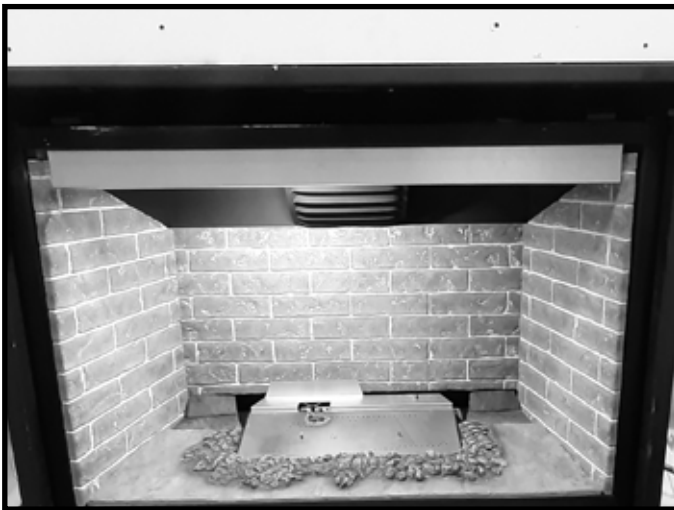
Figure 9 Refractory Kit Installed
