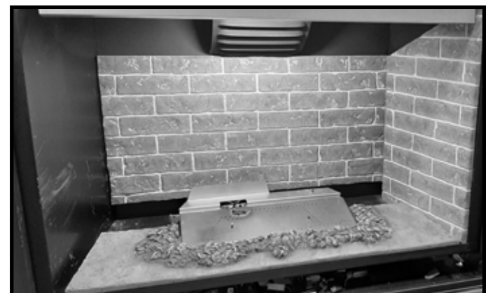
Figure 7 Side Refractory Panel Installed
