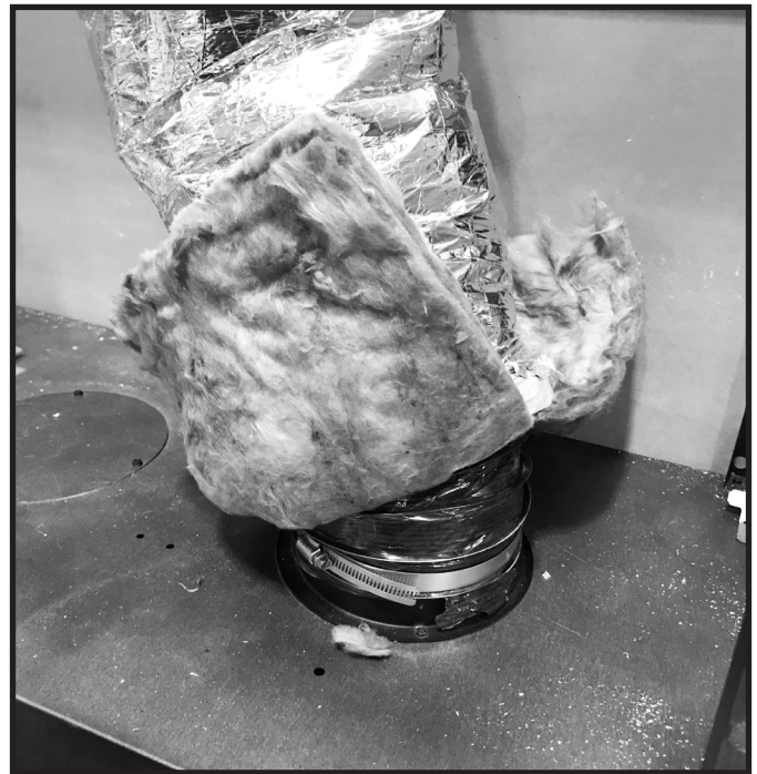
Figure 5.14 Install Flex Venting to Appliance
