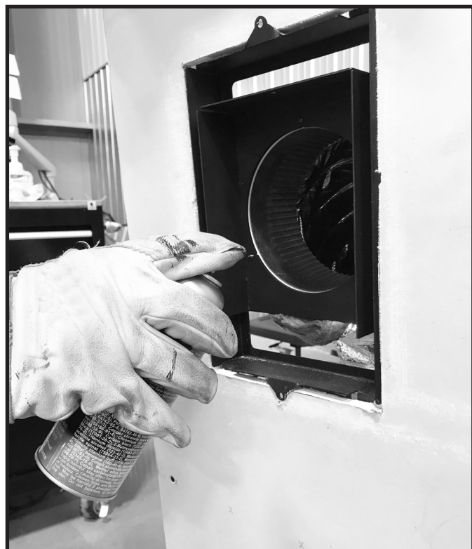
Figure 6.4 Paint Outer Wrapping of Flex Vent (Optional)
