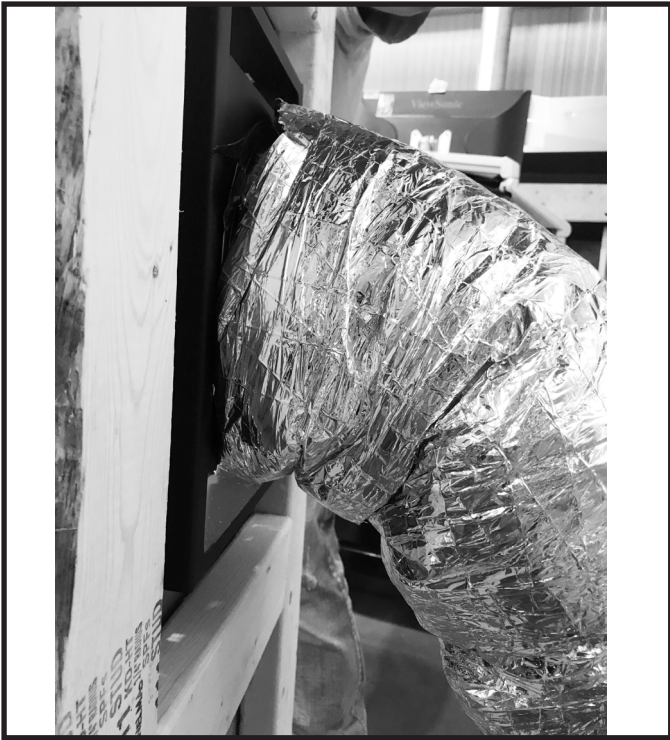
Figure 5.16 Install Flex Venting to Side Discharge Assembly
