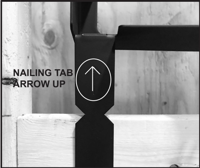
Figure 5.13 Side Discharge Assembly Nailing Tab Orientation
