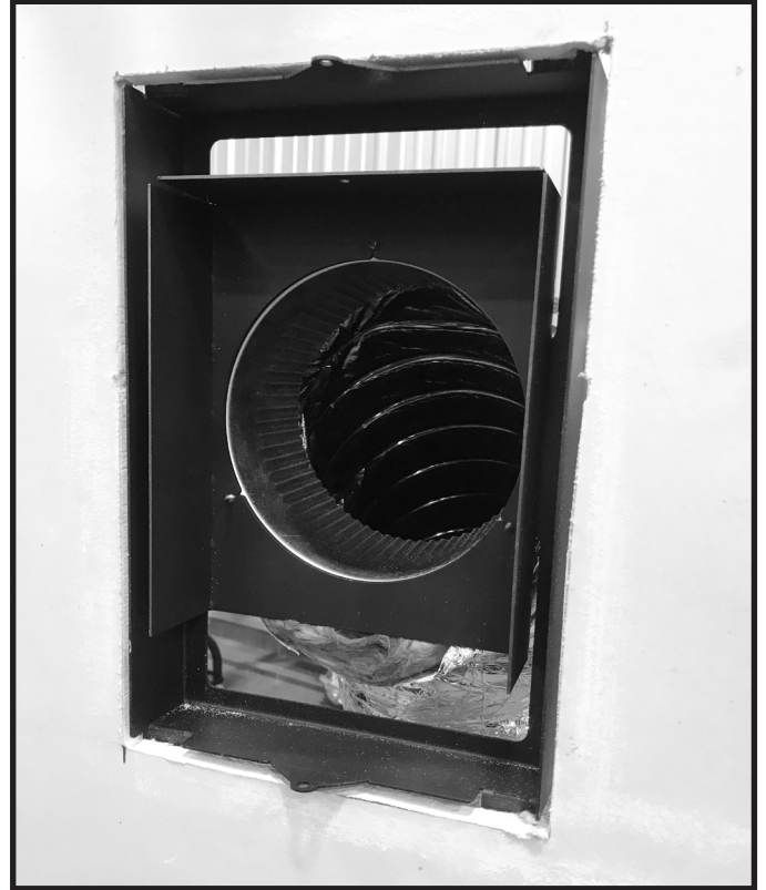
Figure 6.1 Wall Sheathing Installed
