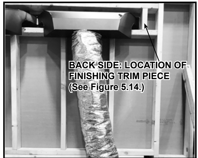
Figure 5.29 Flex Vent Installed with No Kinks
