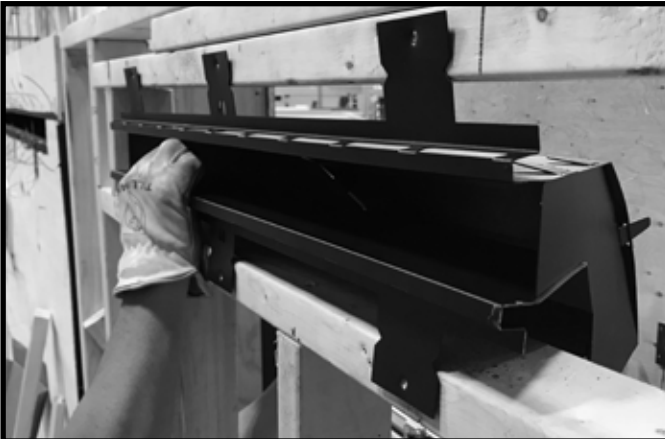
Figure 5.18 Position Plenum
