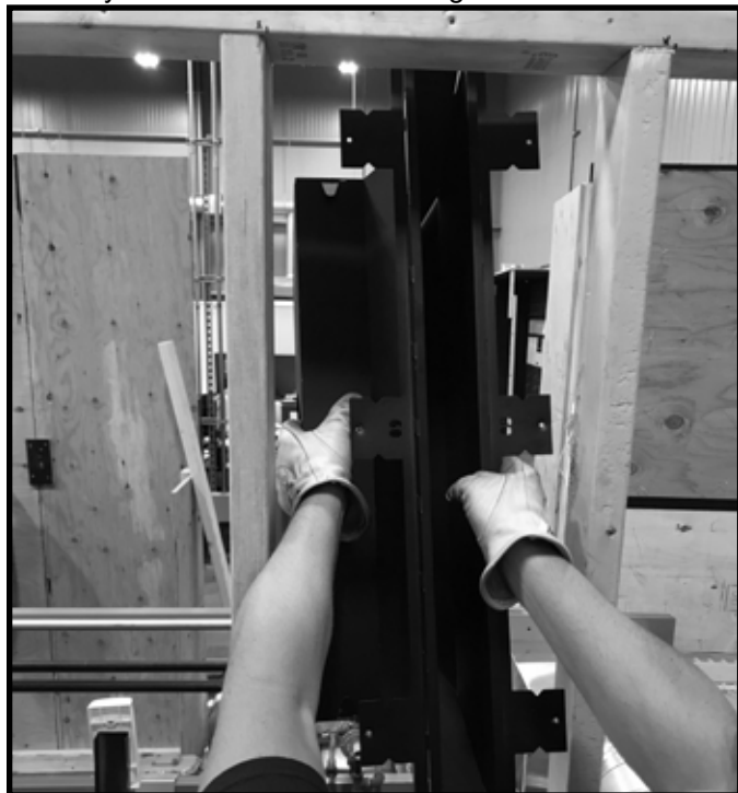
Figure 5.15 Turn Plenum Vertically to Clear Framing Studs
