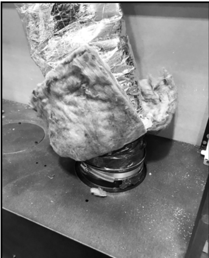
Figure 5.27 Install Flex Venting to Appliance
