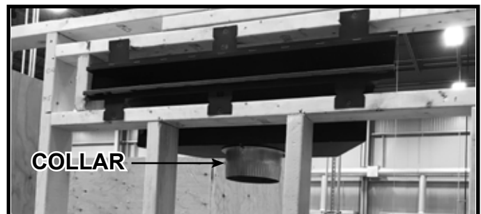
Figure 5.25 Install Collar(s) to Bottom of Plenum
