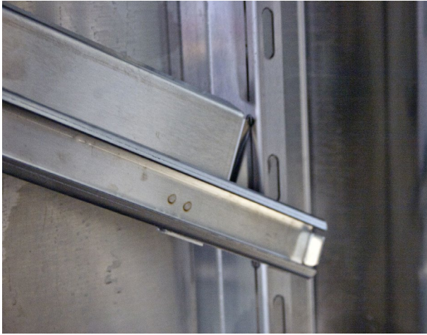
Fig. 14: Set Rail in New Position
