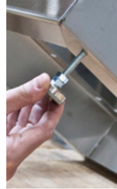
Fig. 8: Insert Leg Leveler into base
