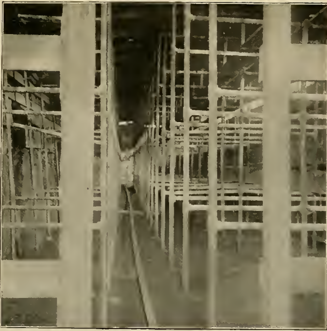
FIG. 1.—A MUSHROOM HOUSE PROVIDED WITH GAS-PIPING FRAMEWORK FOR SHELF BEDS.
