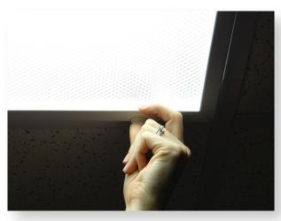
**Step 1:** Open the tabs on your fluorescent light to unlock the frame. (This may require a screwdriver.)
